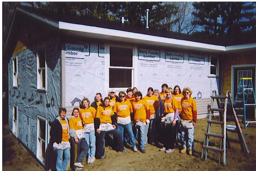
Habitat for Humanity 2005 Ladies' Siding Day
